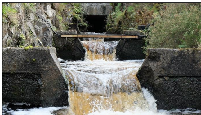
PIT tag antenna located in Loch Doon fish ladder
