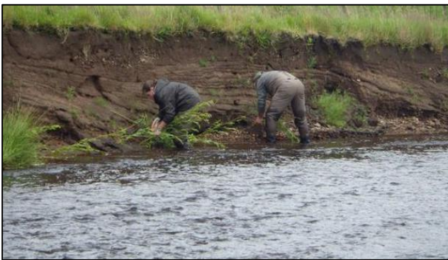
Willow cuttings been plugged into an eroding bank on the upper River Ayr
