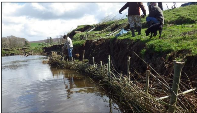
Weaving being constructed, April 2016
