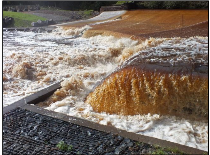
Catrine fish ladder entrance in high water – fish continue to have difficulty finding the entrance.
