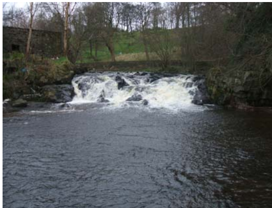
Black Rocks waterfall, Kilmarnock Water, where the plunge pool has been filled and capped with concrete
